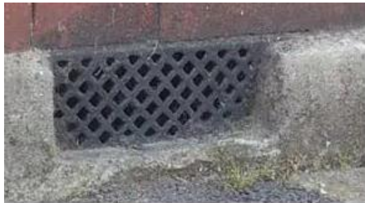
Victorian, ground floor airbrick
