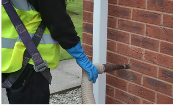
Cavity wall insulation installation. Image: A&M Energy
