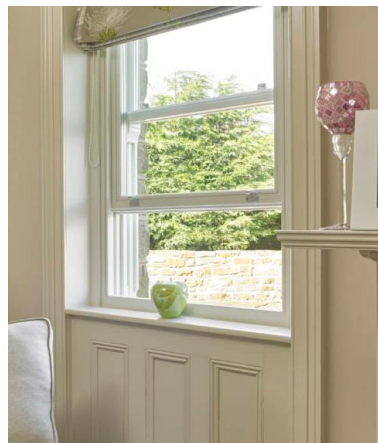
Triple glazed timber sash window in a conservation area. Image: Green Building Store
