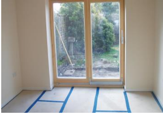
Floating floor above rigid insulation boards Image: AECB
