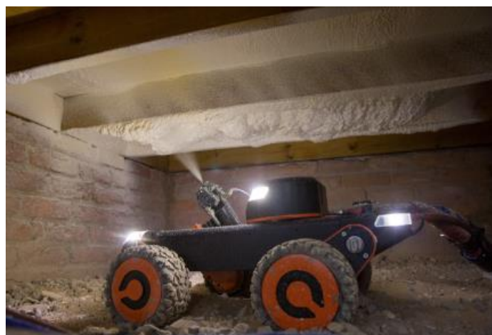
Spray foam insulation using a robot. Image: Energy Saving Trust
