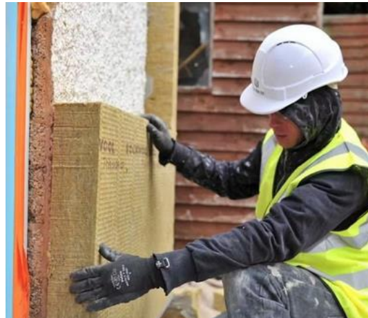
Application of EWI. Image: Rockwool
