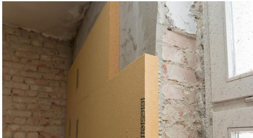
Internal wall insulation. Image: Ecological Building Systems
